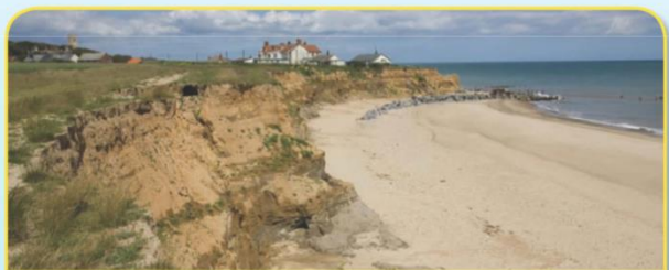
Water loosens and moves sand and rock away from the beach. Areas where grass once grew have been washed away by the water.
